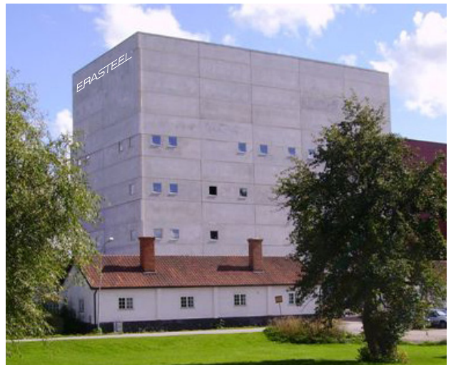
Söderfors Sweden - Durin atomization tower
